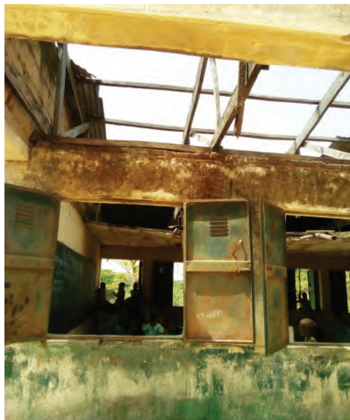
■ A dilapidated structure at the RCM Pilot Science Primary School, Gudi, Akwanga LGA, Nasarawa State
