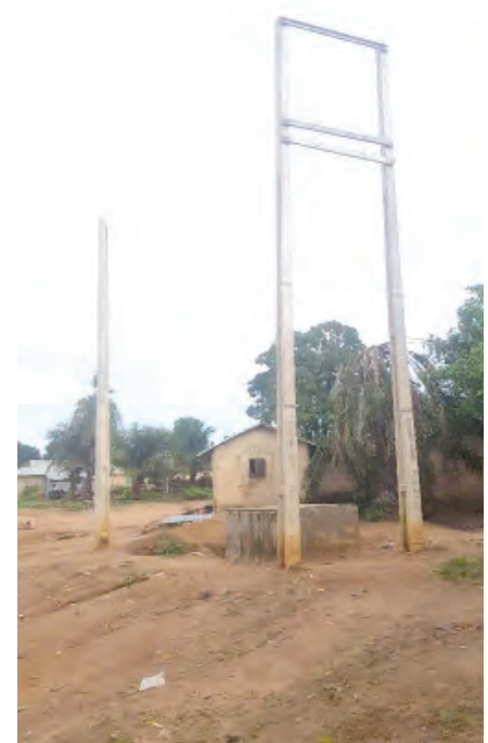
■ These power poles were installed three years ago. They have been abandoned since
