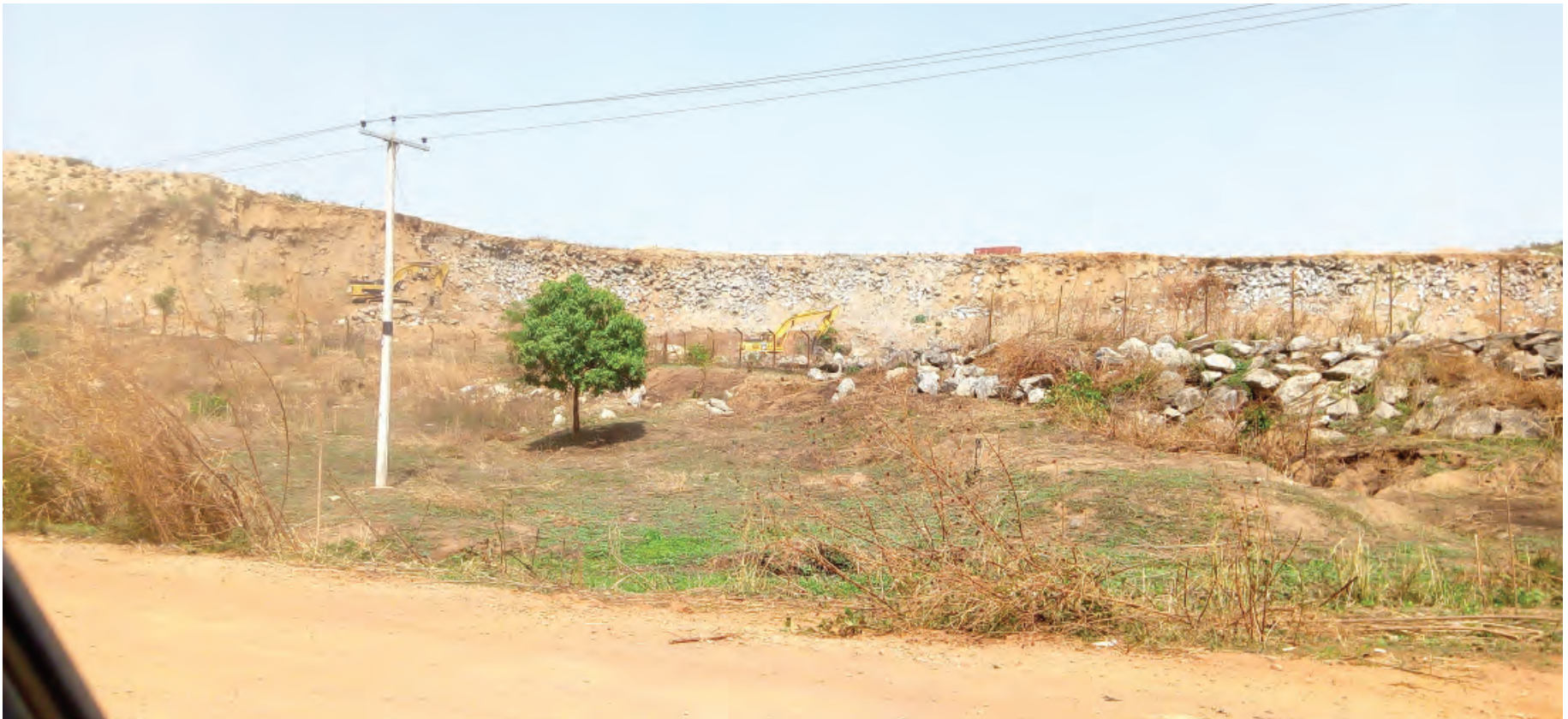
■ Heavy excavation machinies at Mpape mines area
