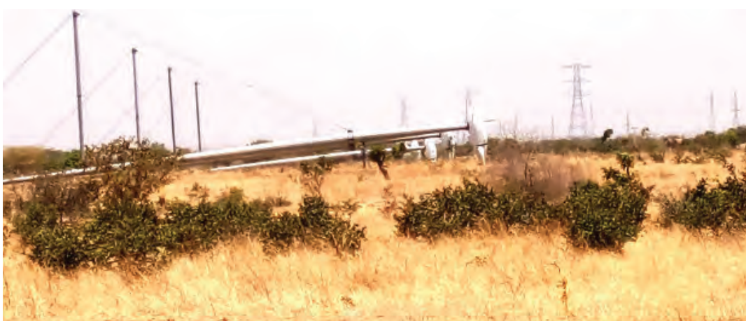
■ The tower laying on the ground
