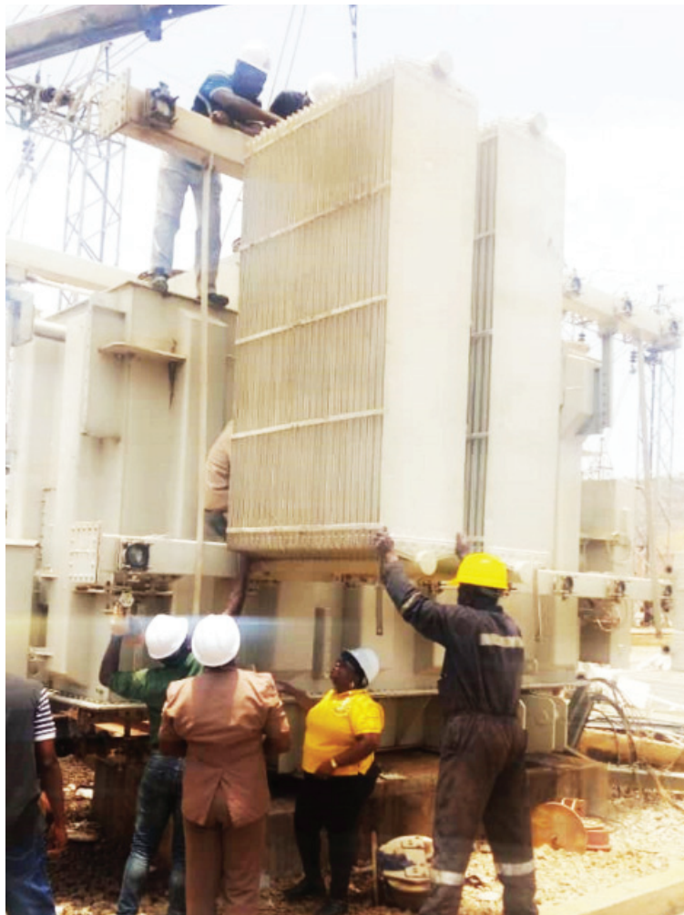
■ TCN crew installing a 60MVA transformer at Kubwa substation, Abuja
