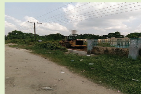
Fig 2.8 On-going fencing at the School of Midwifery, Ituk Mbang, Uruan
