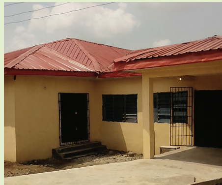
Fig 1.11: Renovated Mortuary of General Hospital Aba, Abia State
