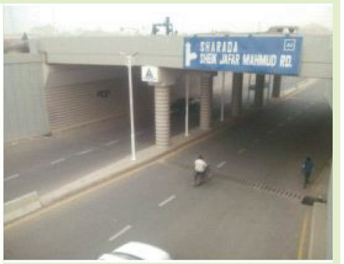
Fig 5.11. under-pass way at Sharada-Pan-shekara
