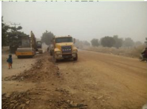
Fig. 5.6. Rehabilitation of Kwanar-Garko Road Rana Road
