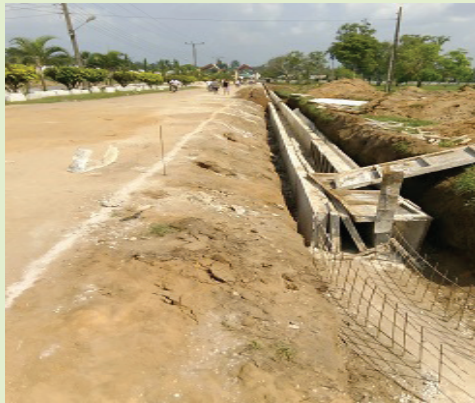
Fig 2.4: On-going drainage construction at College of Education, Afaha Nsit
