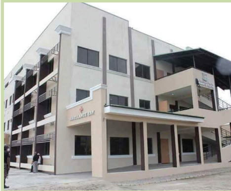
Fig 3.2: Completed diagnostic centre
