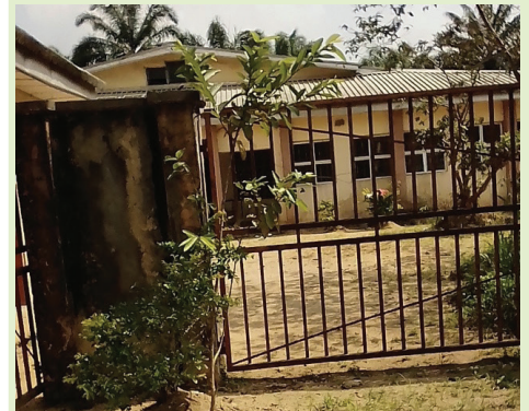
Fig 1.12: Primary Health Centre Otuobi, Umuokiri, Osisioma Local Government,
