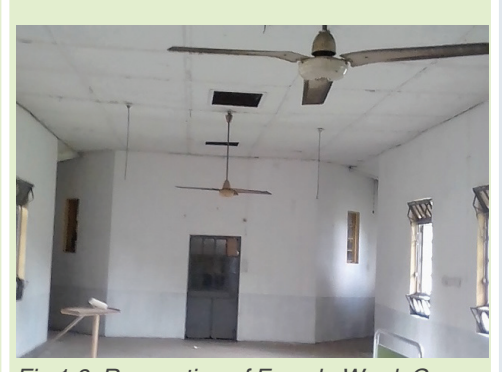
Fig 1.9: Renovation of Female Ward, General Hospital, Aba
