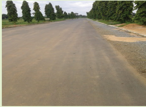
Fig 2.2. Road built during construction of major roads in the state
