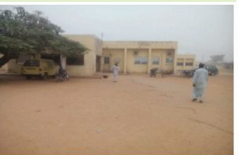
Fig 5.8. Tofa Phc Upgraded To General Hospital
