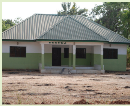
Fig 8 Renovated structure for the Veterinary Clinic being occu
