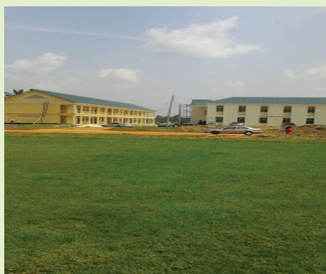
Fig 2.5 Newly completed office and classroom blocks at Akwa Ibom State University, Obio Akpa campus
