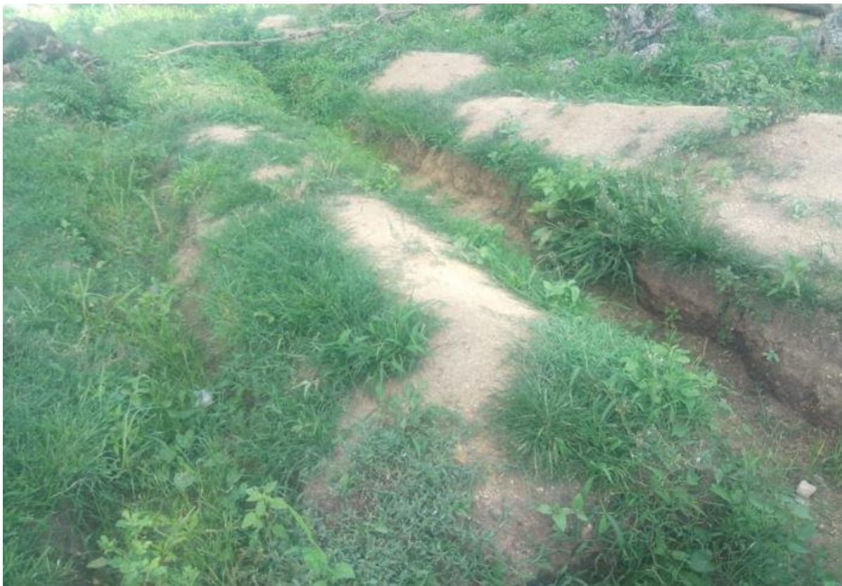
Abandoned foundation of classrooms
